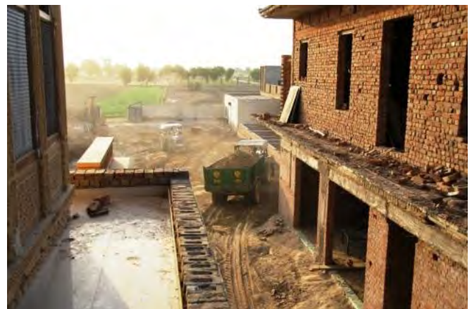
After laying the foundation of the staff residences, tractors haul in dirt to fill in area. The dirt-movers came at dusk and worked some hours in the dark
