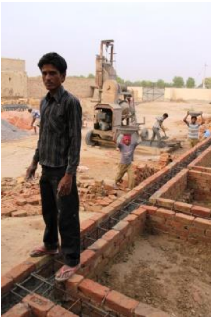
Setting the foundation for our staff residences.
